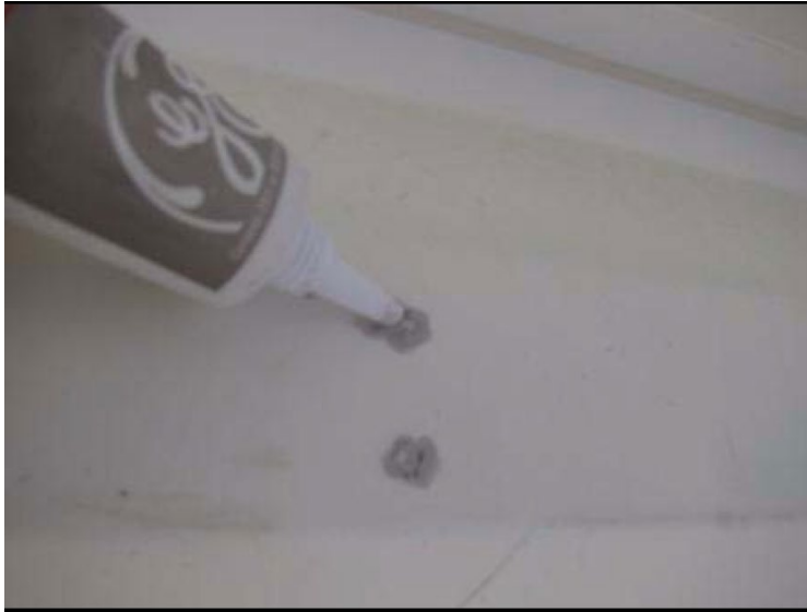
Sealant Applied to Backside
