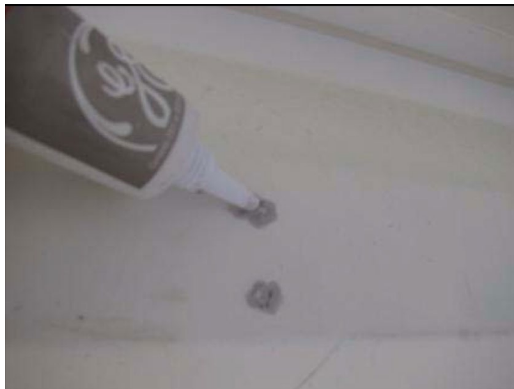
Sealant Applied to Backside
